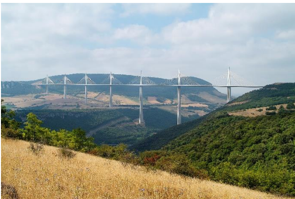
Figure 8: Viaduc de Millau, France. The structure was designed by Michel Virlogeux and Norman Foster, while the execution studies were carried out by the Greisch engineering office — revealing how technical ingenuity and aesthetic vision can converge in a structure that speaks to both function and emotion.
