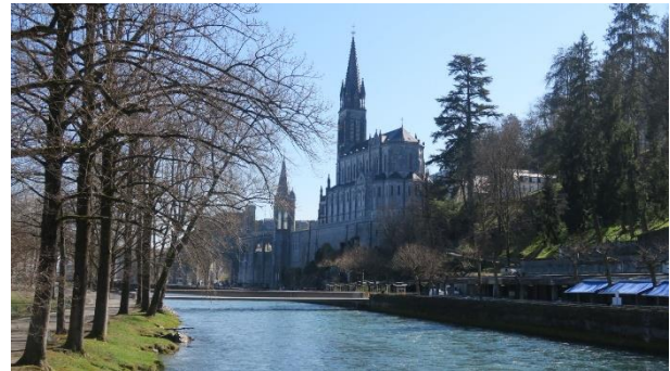
Figure 12: Mobile footbridges over the Gave de Pau, Lourdes. These elegant and functional footbridges serve not only as a means of access, but also as symbols of renewal and accessibility—linking the spiritual and the civic, the local and the universal. A structure designed with purpose and meaning. Arch. Greisch
