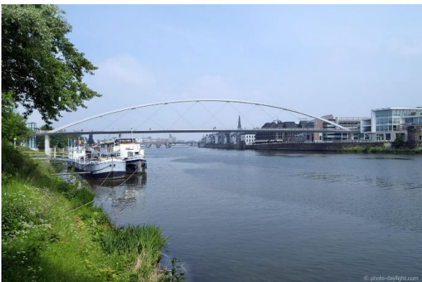
Figure 4 : Hoge Brug, Maastricht. With its slender arch and minimal structure, this pedestrian and cyclist bridge embodies elegance. Every detail serves its function, and nothing is superfluous — demonstrating how a refined use of materials can
