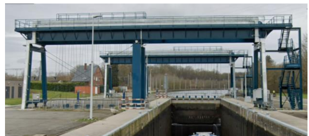
Figure 5. Existing gantry at the Viesville site
