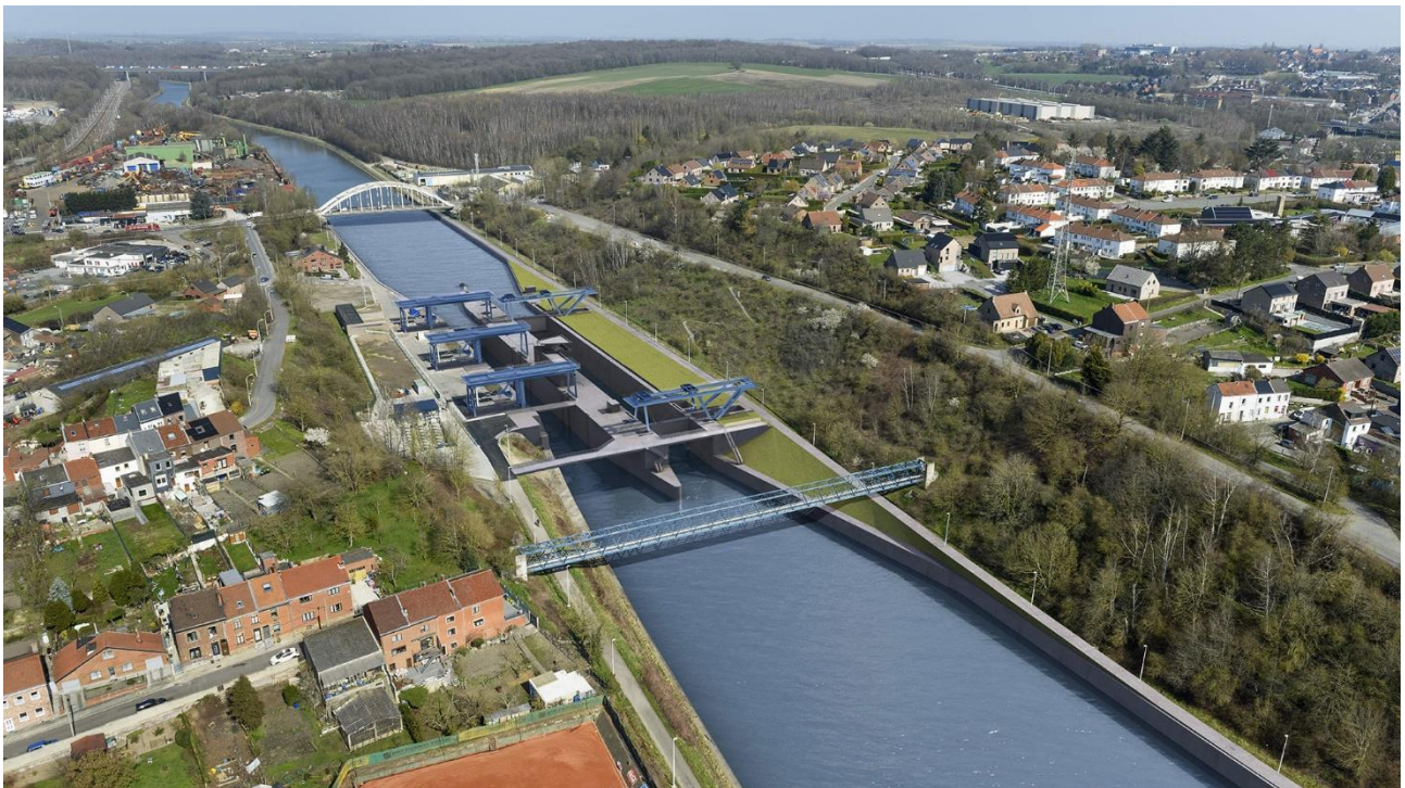
Figure 2. Overview of the Gosselies site
