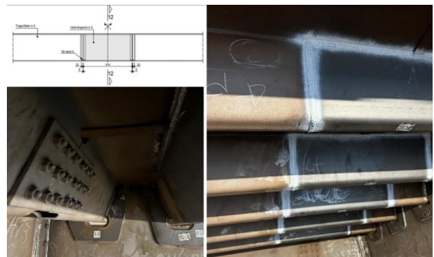
Figure 20: u-rib welded joints
