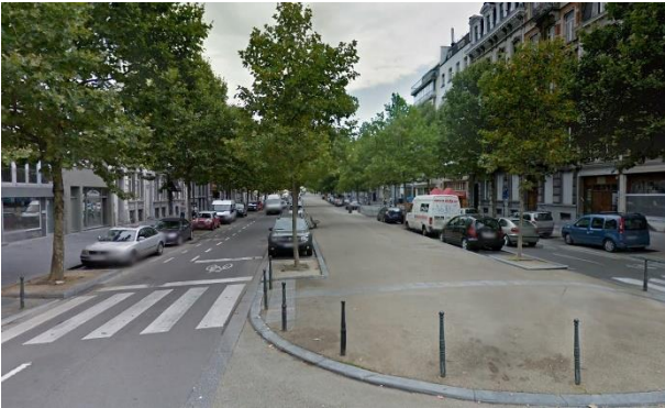
Figure 2. Avenue de Stalingrad before works (photo credit: Google Maps)
