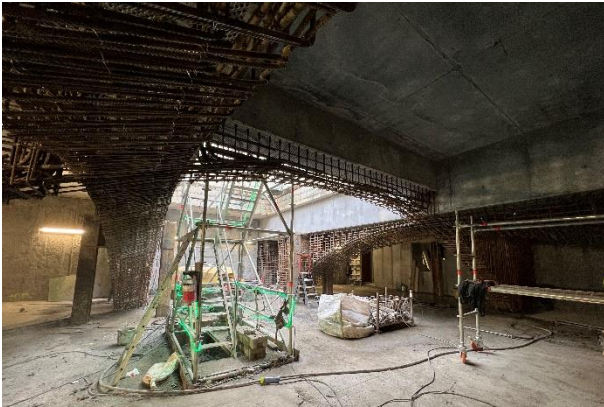
Figure 9. Underground construction of the arches
