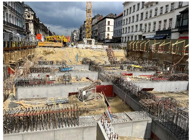
Figure 7. Concreting of the first height of the arch beams completed
