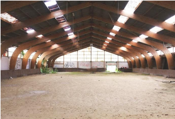
Figure 1. The existing structure in Bierset (BE)
