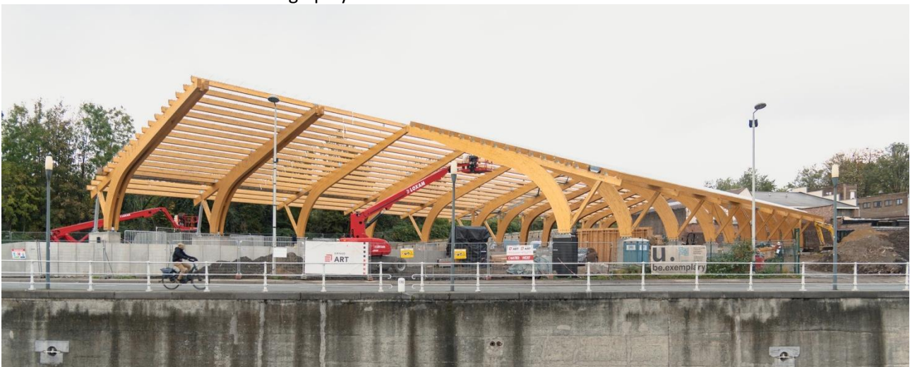
Figure 2. Glulam structure erection in progress
