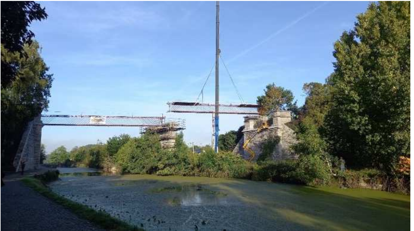
Figure 26: Setting up the second piece between P2 and P3
