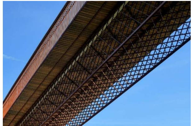
Figure 14: View underside of the deck
