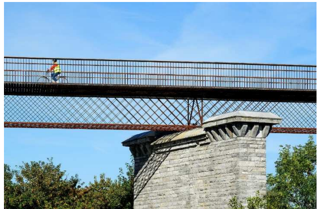
Figure 20 : Zoom on the central support on pier P2
