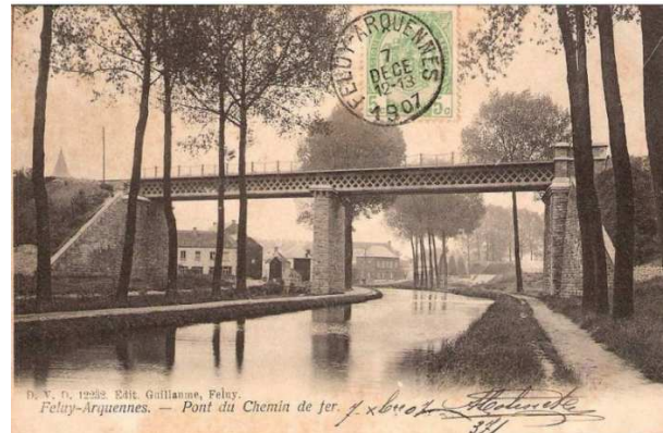
Figure 3: View of the railway bridge before the war 40-45.
