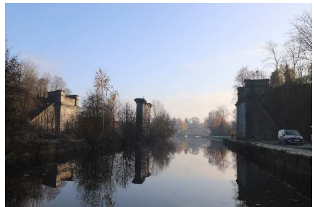
Figure 4: View of the site before the construction of the new footbridge
