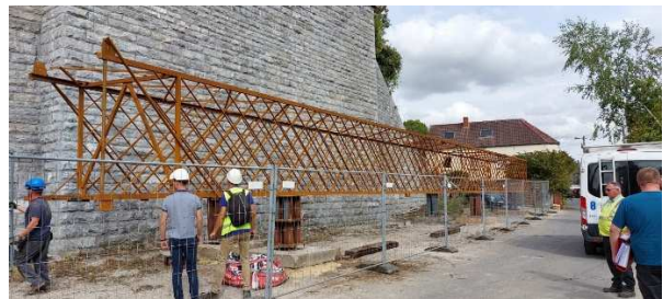
Figure 24: Assembly of the first two sections on site
