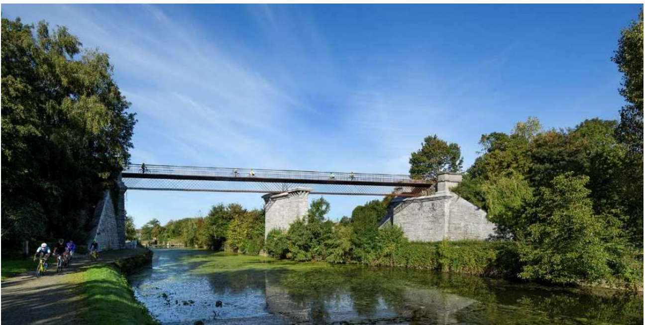
Figure 1: General view of the structure
