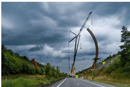
Figure 1. The “Arc Majeur” during erection
